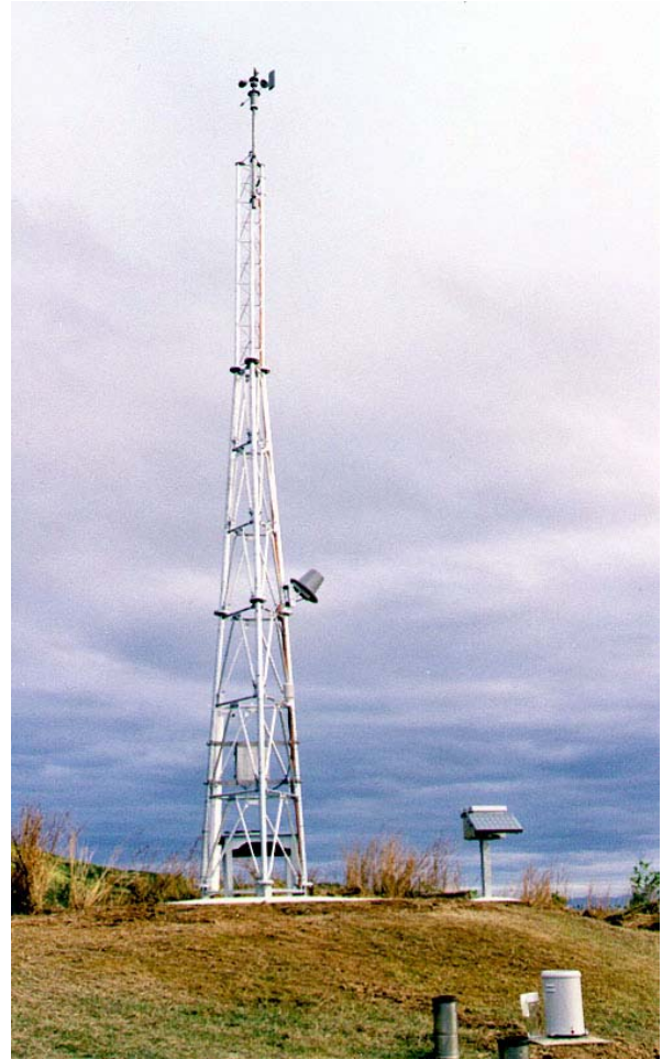
Autonomous SYNOP Station with geostationary satellite transmitter and solar electric power supply.
